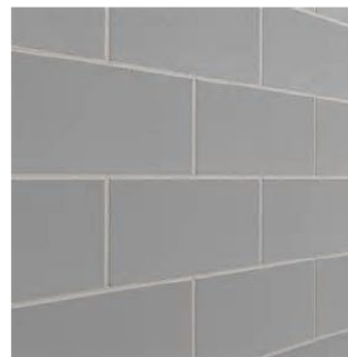
(smooth cmu walls)
